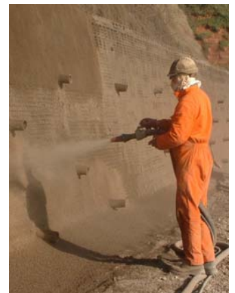
Four of his entries won places - the overall winner was Netting at Shell Cove in the industry category. This excellent photograph captures graphically the efforts by cliff workers installing rock net fixed by soil nails on steep cliffs above the mainline railway near Dawlish. His other winners are below.
