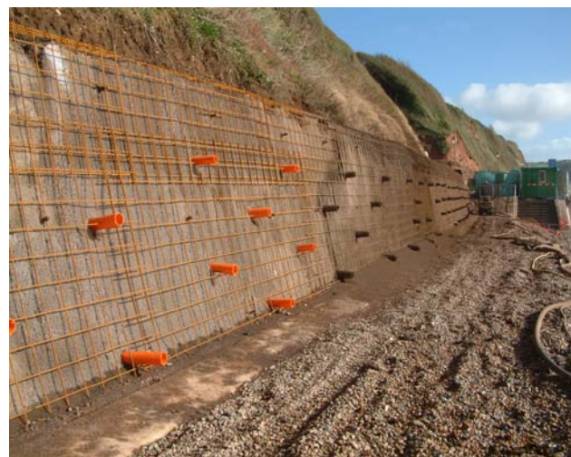
Seaton West Sea Wall where the old sea defence structure has been renovated and faced with sprayed concrete
