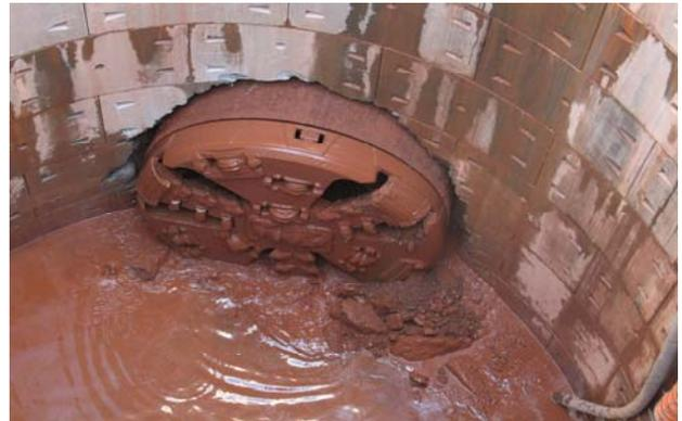
**Tunnel Boring Machine (TBM) emerges into Powderham reception shaft** after its 2km drive under the River Exe estuary to create a gas pipeline tunnel. (photo - D Laming)
